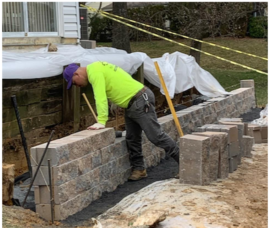
McFall & Berry replace a wall. ▼
